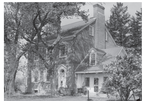
Mordington House in Kent County, Delaware (HABS photo, 1960)
